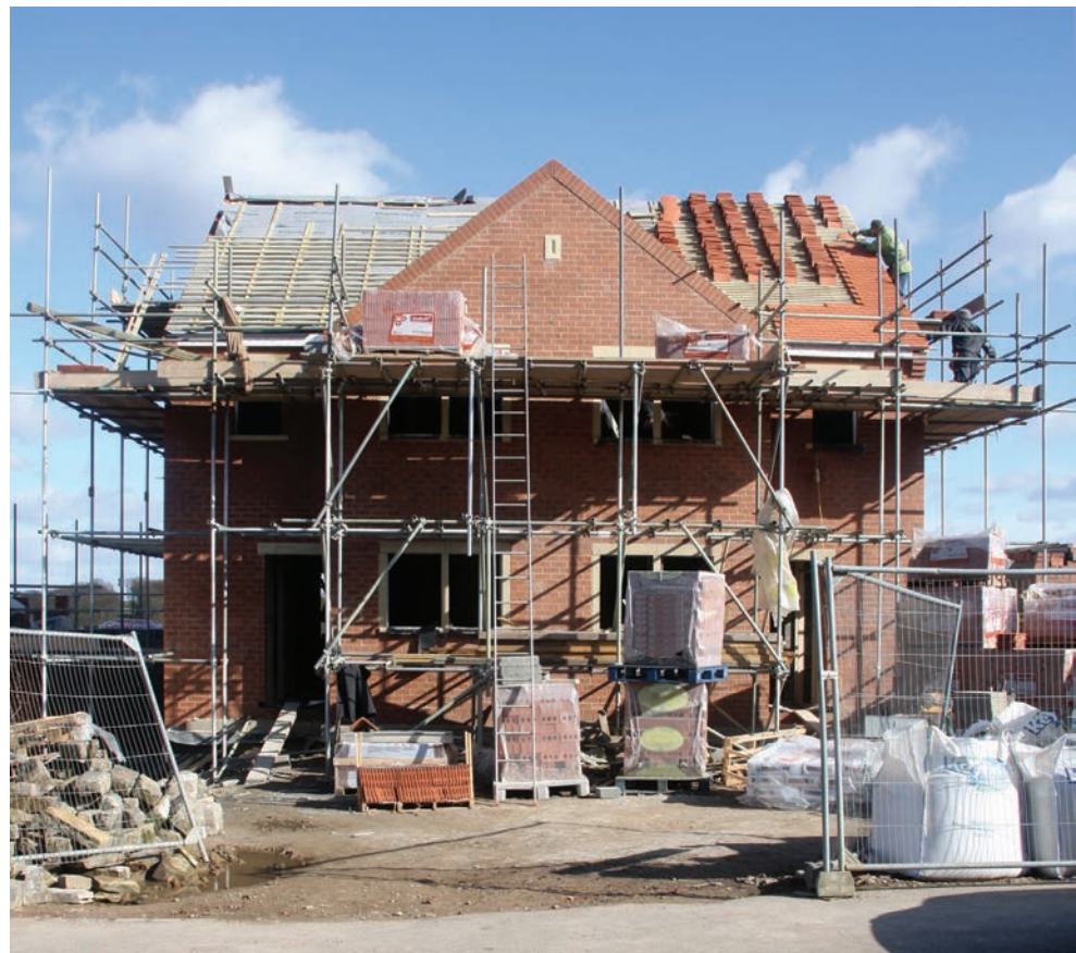
Figure 3.1 Scaffolding and an extension ladder at a building site
