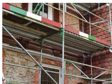
Figure 3.10 System scaffolding
